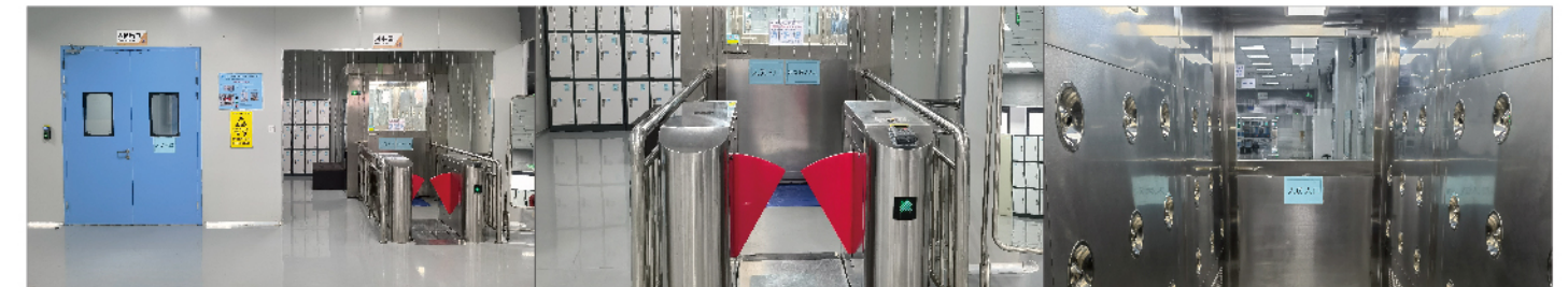
Entrance ESD Detection and Electrostatic Discharge 入口ESD检测及静电释放
